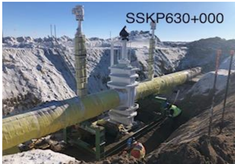
Compaction ongoing MLBV16
