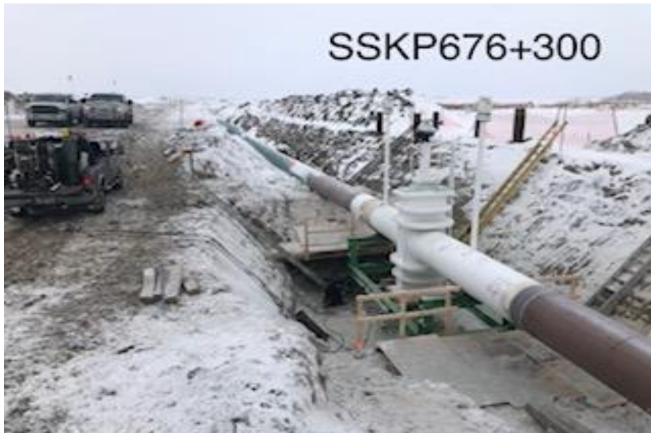
Structural weld MLBV17
