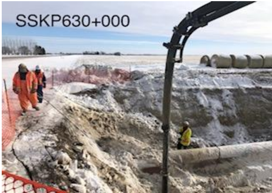
Hydro vac crew removing ice and snow from around MLBV16
