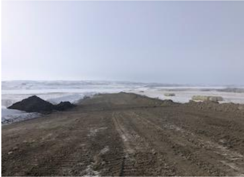
Machine clean completed at water course crossing Chapleau Lake SK WC86
