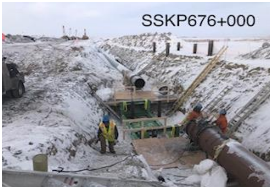
MLBV17 preparation for valve site
